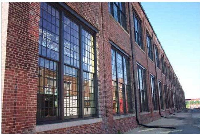
Spencer shops 'Back House' after restoration
